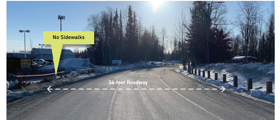
Fig. 73: Existing States Avenue at Soldotna Creek Park (2023)
