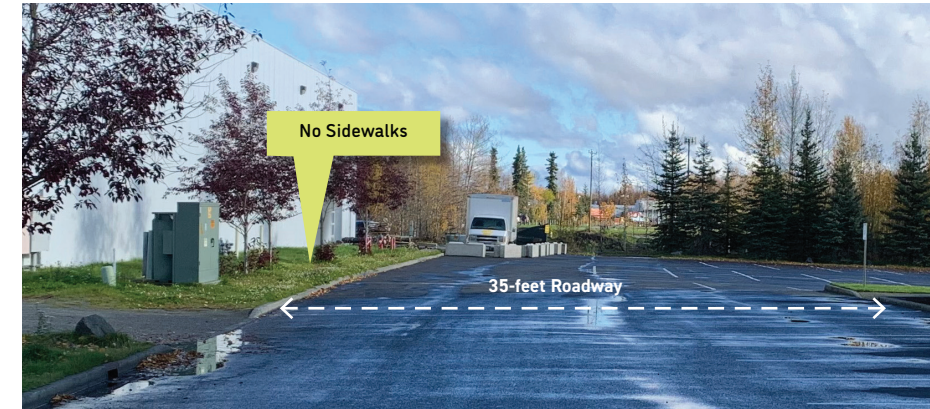
Fig. 71: Existing Driveway at Aspen Hotel (Looking Northeast)
