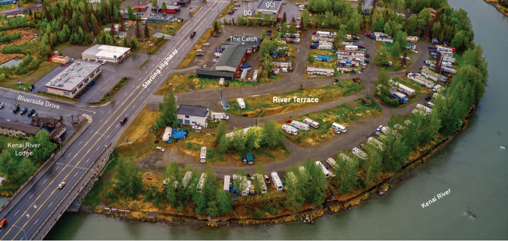
Fig. 104: Existing riverfront property (2023)
