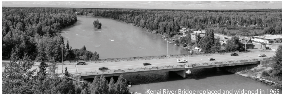
Kenai River Bridge replaced and widened in 1965
