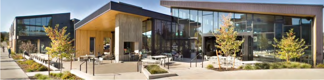
The Grove Market Hall – Bend, Oregon credit: Hacker Architects
